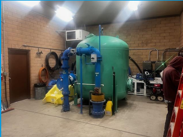
Raw water comes from Intake PS into Clarifier
